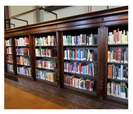
Fully adjustable, metal cantilever shelving was installed inside the original wooden cubbies where the damaged wooden shelves were removed.
